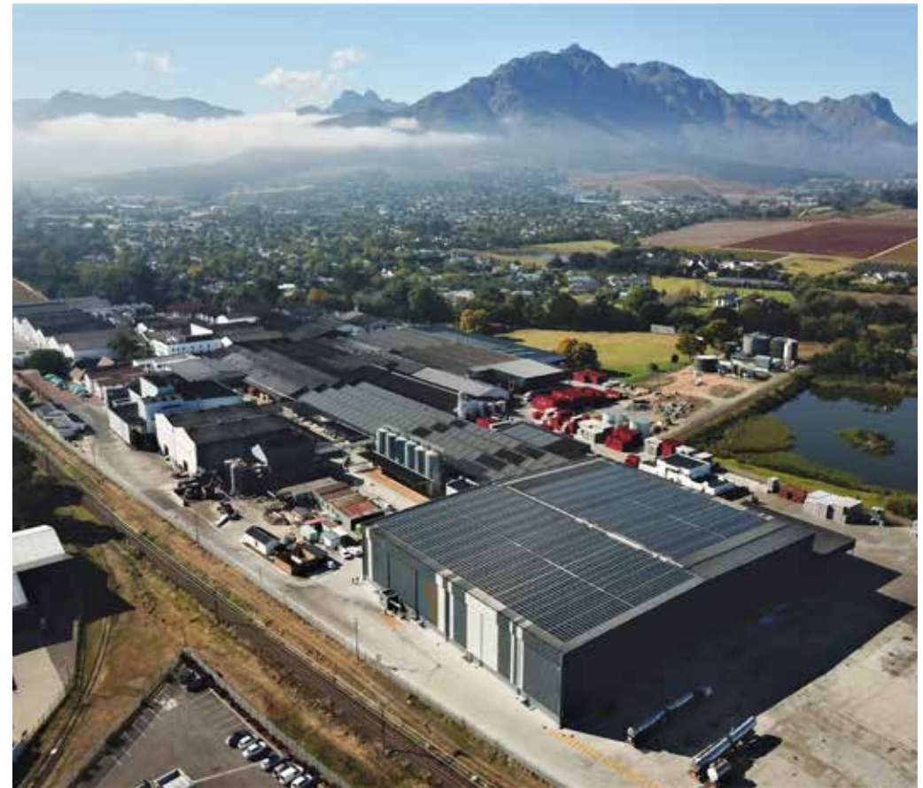
SOLAR POWER INSTALLED BY TFS IN 2021 FOR AN INDUSTRIAL CLIENT IN SOUTH AFRICA
